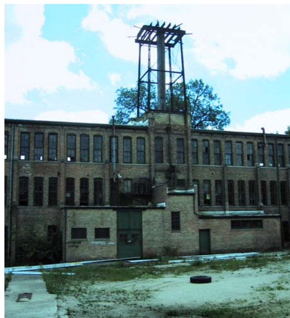
Rear view, Chester St. side of the facility, July 2010
