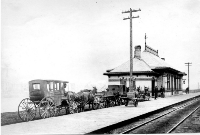
The railroad comes to Elgin in 1850 and depots are built on the east and west sides of town.
