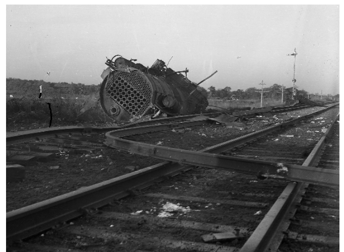
The Overturned Boiler Amid Twisted Rails (cn2359)
